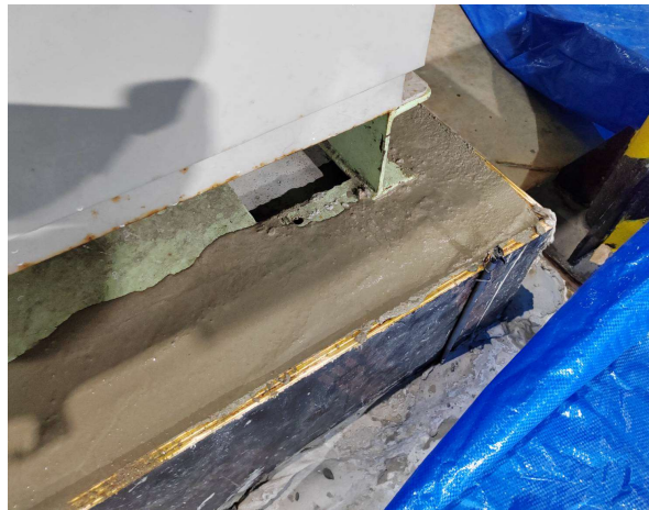
2. Repairing the concrete foundation
