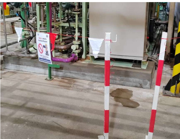
3. Repairing the foundation finished
