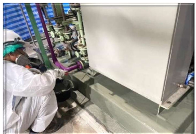
Repairing foundation
