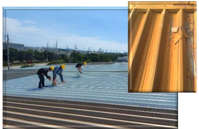
Repainting on a roof
