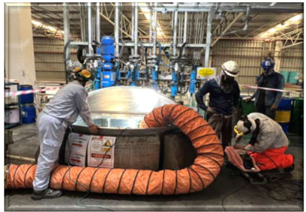
Cleaning inside tank
