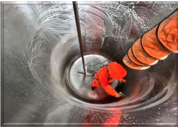
Cleaning inside tank
