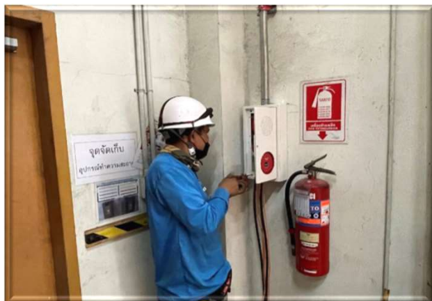
Checking the fire alarm system
